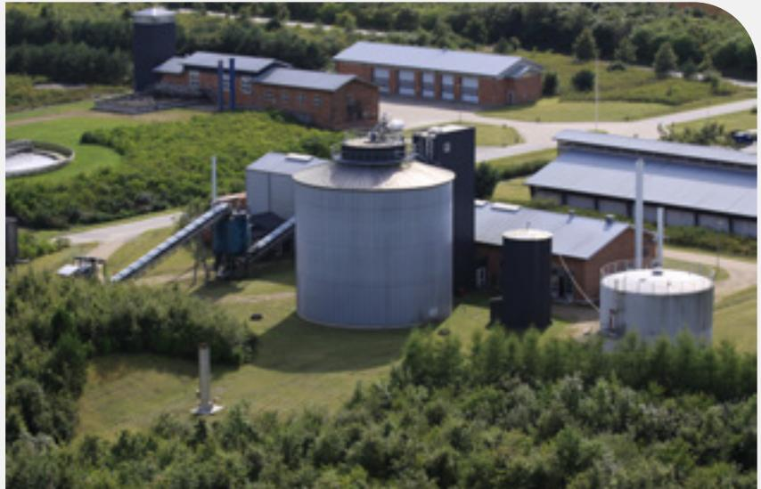
To address these issues, Veolia Water Technologies has developed the ANITA™ Mox solution, an alternative to conventional nitrification/denitrification processes for treating effluents with a high ammonia concentration. ANITA™ Mox can treat this sidestream nitrogen load without any additional source of carbon while reducing the electric power consumption by 60%.
